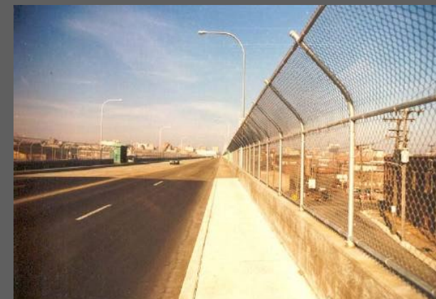
IS a freeway overpass
